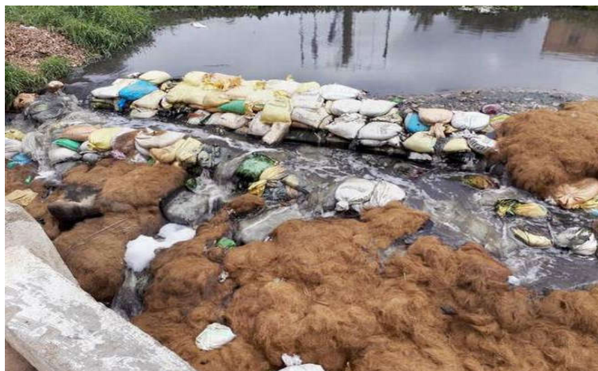
Fig. 12. Coir blocks placed at the weir of lake to suppress frothing
