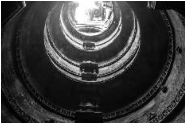
Fig.6.2.2 Circular Well at Dada Harir Stepwell, Gujarat
