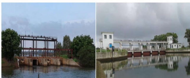
Fig. 9. The Guidel dam (left) and Affiniam dam (right)
