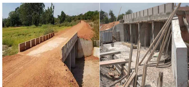
Fig.11. Heir dam at Cabrousse under construction
